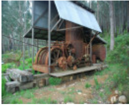
WASHINGTON WINCH SOHE 2008
