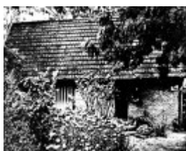
76 - Pise House Langi Dorn 4 Fay St - Shire of Eltham Heritage Study 1992
