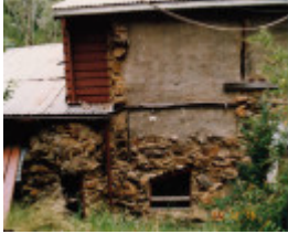
Stonygrad House Hamilton Rd Colour - Shire of Eltham Heritage Study 1992
