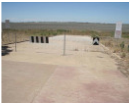
H2208 Boga Slipway Feb 09 PM2
