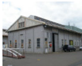
Before Photograph - Reference F3916 2014
