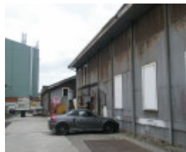
Before Photograph - Reference F3916 2014
