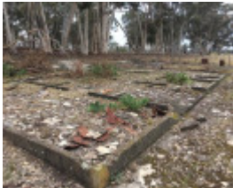
2017_Concrete floor slabs_F8.jpg
