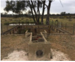
2017_Water treatment plant_F4.jpg
