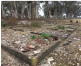
2017_Concrete floor slabs_F8.jpg
