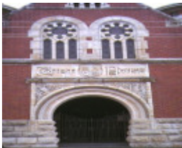
bairnsdale courthouse nicholson street bairnsdale entrance detail
