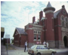
bairnsdale courthouse nicholson street bairnsdale tower view
