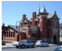
H1462 Bairnsdale Court House from the SW
