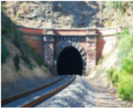
big hill railway precinct bendigo coliban system water race apr1998
