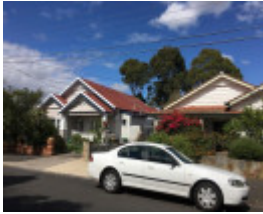
Hickford Street Precinct
