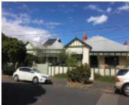
Hickford Street Precinct
