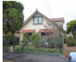
Hickford Street Precinct
