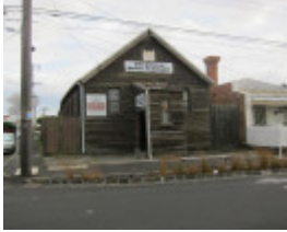
Church (former), 170 Albert St Brunswick
