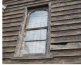
Church (former), 170 Albert St Brunswick
