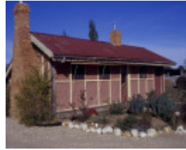
h00839 1 powell's prefabricated house main rd campbells creek front exterior
