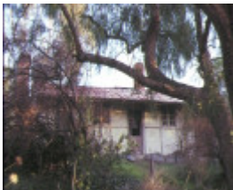
powell's prefabricated house main road campbells creek rear view
