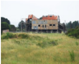
WONTHAGGI STATE COAL MINE CENTRAL PRECINCT SOHE 2008
