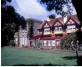
h00289 1 murndal murndal road hamilton homestead
