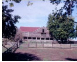
h00289 murndal murndal road hamilton woolshed
