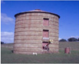
h00289 murndal murndal road hamilton silo
