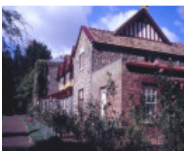
h00289 murndal murndal road hamilton homestead close up
