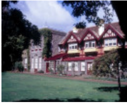
h00289 1 murndal murndal road hamilton homestead
