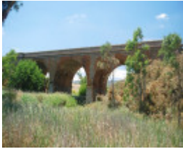
RAIL BRIDGE SOHE 2008
