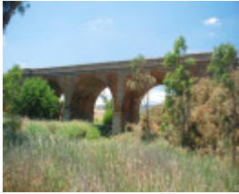
RAIL BRIDGE SOHE 2008
