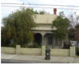
House - 232 Victoria Street, Brunswick
