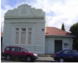
Coburg Court House
