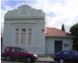
Coburg Court House
