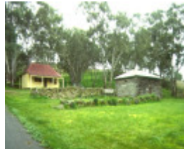
h306 log lockup harrow july 1995
