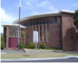
St Bernard's Catholic Church - 10-38 Patterson Street, COBURG,
