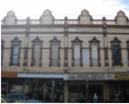
Dunne's Building - 436-442 Sydney Road, Coburg
