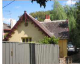
FORMER INVERGOWRIE LODGE SOUTH ELEVATION
