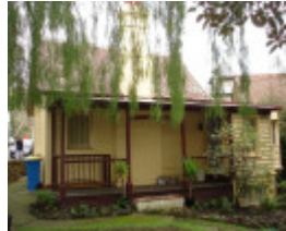
H0517 facade from Burwood Road
