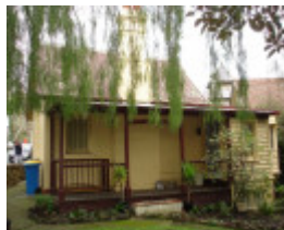
H0517 facade from Burwood Road
