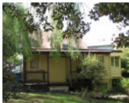
FORMER INVERGOWRIE LODGE NORTH ELEVATION
