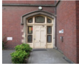
H0516 FORMER ES&A BANK (MANRESA PEOPLE'S CENTRE) LHA 2015 6.JPG
