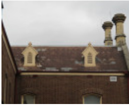
H0516 FORMER ES&A BANK (MANRESA PEOPLE'S CENTRE) LHA 2015 4.JPG
