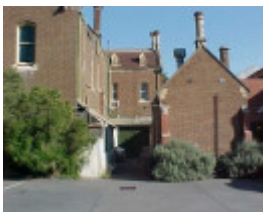
H00516 former es a bank rear elevation 2003
