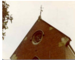
former es&a bank burwood road hawthorn roof detail 1977
