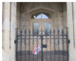
H0516 FORMER ES&A BANK (MANRESA PEOPLE'S CENTRE) LHA 2015 3.JPG
