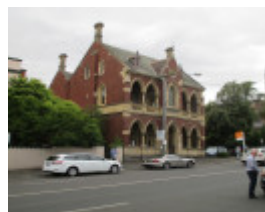
H0516 FORMER ES&A BANK (MANRESA PEOPLE'S CENTRE) LHA 2015 2.JPG
