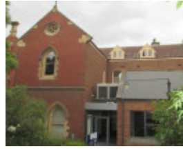
H0516 FORMER ES&A BANK (MANRESA PEOPLE'S CENTRE) LHA 2015 5.JPG
