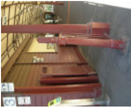
Painted cast iron and timber fence and gate components beneath the northern end of the Platform 2 and 3 canopy
