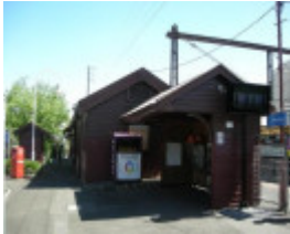
Northern ends of east [Platform 1] buildings viewed from the Evansdale Rd footpath
