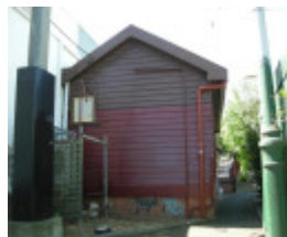
Platform 1 building - southwest elevation
