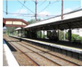
HAWTHORN RAILWAY STATION COMPLEX SOHE 2008
