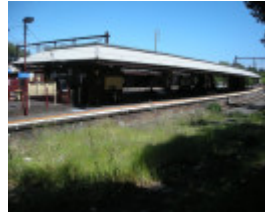
Looking at Platform 3 from the north, with the entire Platform 2 and 3 canopy visible
