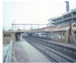
hawthorn railway station end view
