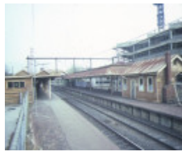
hawthorn railway station end view
