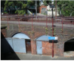
The northern-most of the arched alcoves beneath the pedestrian walkway have been enclosed to create storage areas
