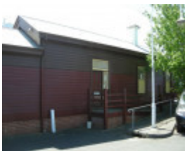
Southeast elevation of the Platform 1 building viewed from the carparking area
