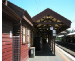
Looking southward along Platform 1 at its buildings and canopy - the canopy timber king-post trusses and support brackets of bent rail are visible
