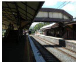
Looking northwards along the edge of Platform 2 with the south elevation of the roofed footbridge between the Platforms visible at upper right
