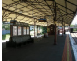
Looking north from the mid-point of the edge of Platform 2 - the Station nameboard and back-to-back timber benches in foreground are significant elements
