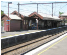
HAWTHORN RAILWAY STATION COMPLEX SOHE 2008
