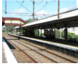
HAWTHORN RAILWAY STATION COMPLEX SOHE 2008
