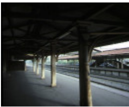
hawthorn railway station platform detail
