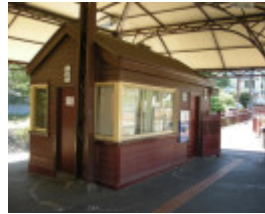
Small building under the northern end of the Platform 2 and 3 canopy
