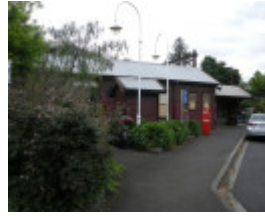
Platform 1-side buildings viewed from the south on Evansdale Rd
