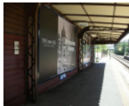
Looking south beneath the Platform 1 cantilever-truss canopy
