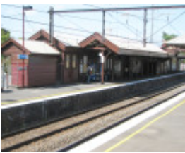
HAWTHORN RAILWAY STATION COMPLEX SOHE 2008
