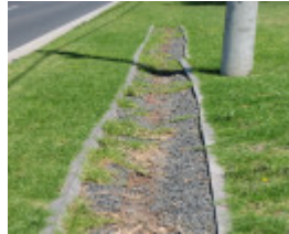
MARKET GARDENERS TRAM PLATEWAY SOHE 2008
