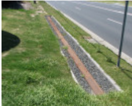
MARKET GARDENERS TRAM PLATEWAY SOHE 2008
