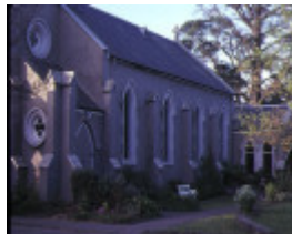
st johns anglican church heidelberg side view
