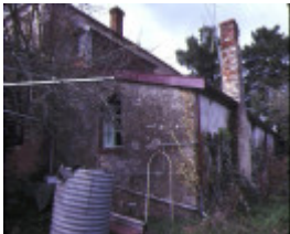
former macaroni factory main rd hepburn springs rear view sep1981
