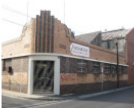
Steel Company of Australia (former) - 14 Frith St. Brunswick
