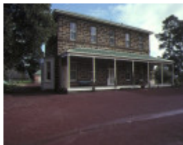
1 mt talbot homestead mt talbot horsham homestead front elevation sep1979
