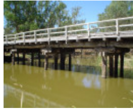
h01850 1 danns bridge over bet bet creek dunolly eddington road eddington close view she project 2004
