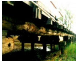
h01850 danns river bridge ntv
