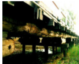
h01850 danns river bridge ntv
