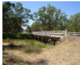
h01850 danns bridge over bet bet creek dunolly eddington road eddington long view she project 2004
