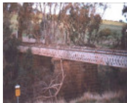
1 glenmona river bridge ntv
