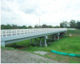
BAYLES BRIDGE NO.1 & 2 SOHE 2008
