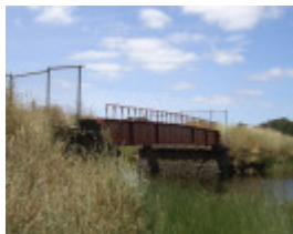
HOTSPUR BRIDGE SOHE 2008
