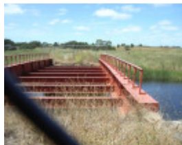
HOTSPUR BRIDGE SOHE 2008
