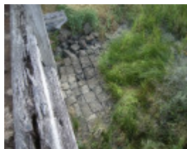
BURCHETT CREEK BRIDGE SOHE 2008
