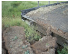
BURCHETT CREEK BRIDGE SOHE 2008
