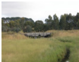
BURCHETT CREEK BRIDGE SOHE 2008
