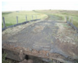
BURCHETT CREEK BRIDGE SOHE 2008
