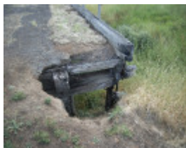
BURCHETT CREEK BRIDGE SOHE 2008
