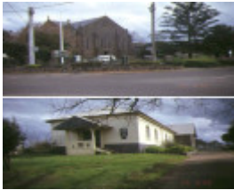
1 st stephens church and school portland
