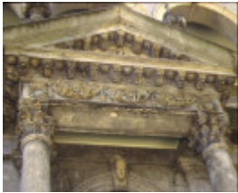
ravenswood ivanhoe detail of stonework
