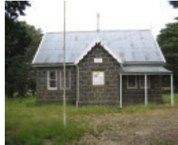
Former Leigh Shire Hall
