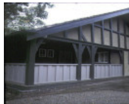
Waller house detail of front verandah
