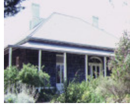
1 strathulloh homestead melton south front view of homestead
