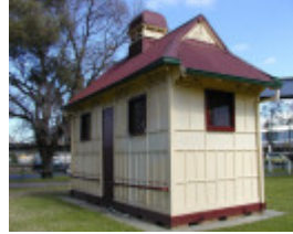
former grand rank cabman's shelter near footbridge yarra park jolimont side she project 2004
