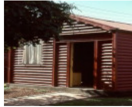
1 bellhouse iron house
