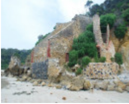
WALKERVILLE LIME KILNS SOHE 2008
