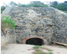
WALKERVILLE LIME KILNS SOHE 2008
