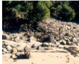
h02043 walkerville jetty timbers 2003
