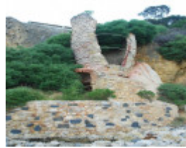
WALKERVILLE LIME KILNS SOHE 2008
