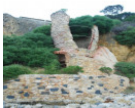
WALKERVILLE LIME KILNS SOHE 2008
