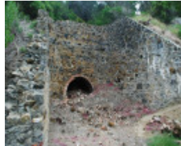
WALKERVILLE LIME KILNS SOHE 2008
