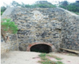
WALKERVILLE LIME KILNS SOHE 2008
