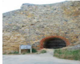
WALKERVILLE LIME KILNS SOHE 2008
