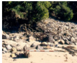
h02043 walkerville jetty timbers 2003
