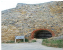
WALKERVILLE LIME KILNS SOHE 2008
