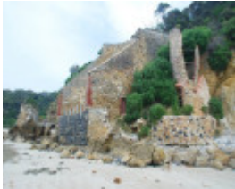
WALKERVILLE LIME KILNS SOHE 2008
