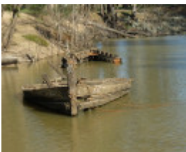
20151005_Echuca wharf Wet Dockand B22 Barge 15.JPG
