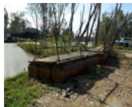
20151005_Echuca wharf Wet Dockand B22 Barge 4.JPG
