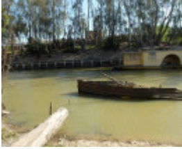
20151005_Echuca wharf Wet Dockand B22 Barge 6.JPG
