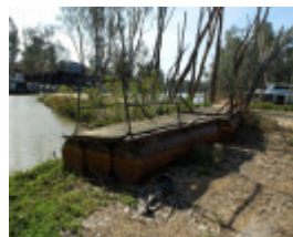
20151005_Echuca wharf Wet Dockand B22 Barge 4.JPG
