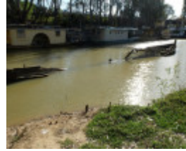
20151005_Echuca wharf Wet Dockand B22 Barge 8.JPG
