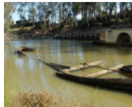
20151005_Echuca wharf Wet Dockand B22 Barge 10.JPG
