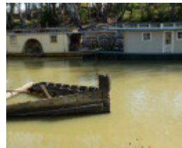
20151005_Echuca wharf Wet Dockand B22 Barge 11.JPG
