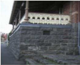
former police station ballarat detail of verandah
