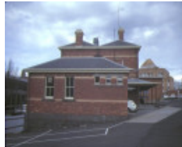
former police station ballarat side elevation
