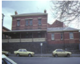
former police station ballarat rear view
