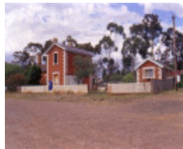
Kangaroo Flat Railway Station Complex Street Elevation
