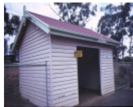
kangaroo flat railway station complex outbuilding jul1984
