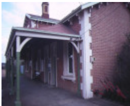
kangaroo flat railway station complex platform view jul1984
