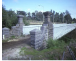
1 iron bridge maribyrnong river front view sep1984
