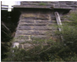
iron bridge maribyrnong river stone support detail
