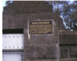
iron bridge maribyrnong river plaque detail
