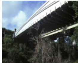
iron bridge maribyrnong river side elevation sep1984
