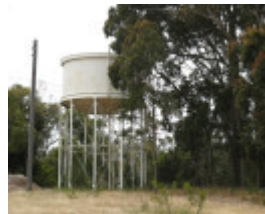
Westerfield_Frankston_elevate water tank_KJ_Dec 08
