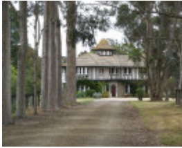
Westerfield_house from drive_KJ_Dec 08
