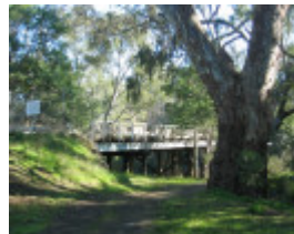
h00092 ol goulburn riv bridge seymour july 05 setting
