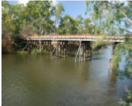
OLD GOULBURN RIVER BRIDGE SOHE 2008
