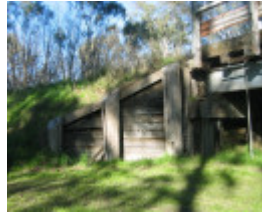
h00092 ol goulburn riv bridge seymour july 05 abutment
