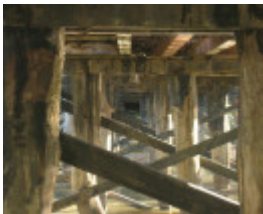
h00092 ol goulburn riv bridge seymour july 05 trestles
