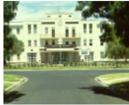
Former Mildura Base Hospital Main Entrance 2001
