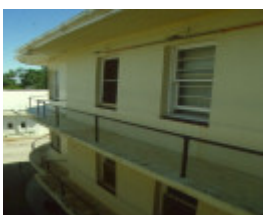
Former Mildura Base Hospital West Wing 2001
