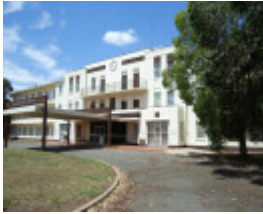
FORMER MILDURA BASE HOSPITAL SOHE 2008
