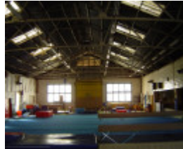
6168 Warragul Drill hall may07 ac 16
