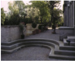
ross house kew front steps detail
