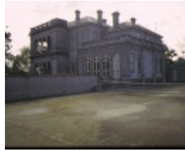
ross house kew rear view
