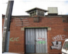
City of Brunswick Electricity Supply transformer station (former) - Howarth Street, Brunswick
